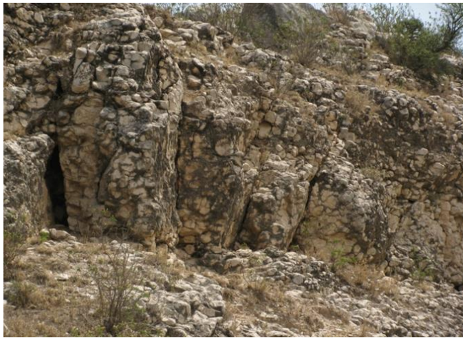
Fig4: Orientation of bedding and joints (Mostly joints are dip joint)
